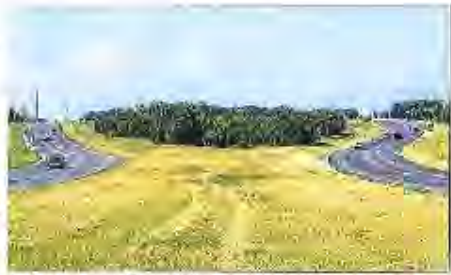
The Texas Department of Transportation aims to build MoPac lanes underpass at Slaughter and La Crosse. TxDOT estimates that two to three years of construction on the project, which is already fully funded by the agency, would commence by late spring 2015. www.txdot.gov
